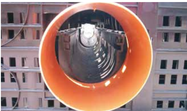
Opening for camera inspection
