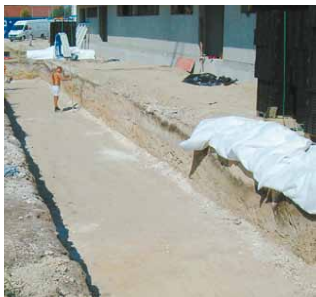
Building pit with granular sub-base
