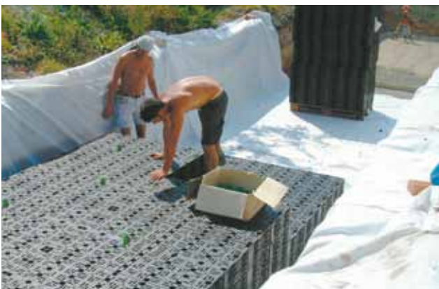
Laying several layers with connection adapter
