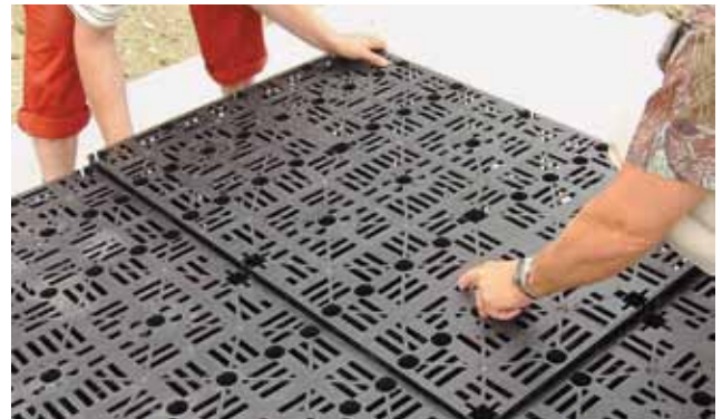
C Engage the connector hooks by lifting the block slightly and moving the longer side against the side of the block already laid.
