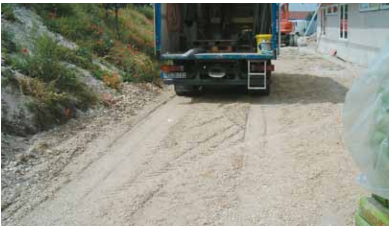
When the covering layer has reached a thickness of 50 cm it can support HGV of 12 t gross vehicle weight rating.
