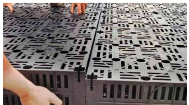
D Lower the DRAINFIX BLOC again and both sides of the block will be securely linked with resistance against thrust.
